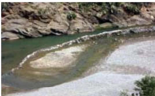
**Small-scale water weir built by a traditional method**
