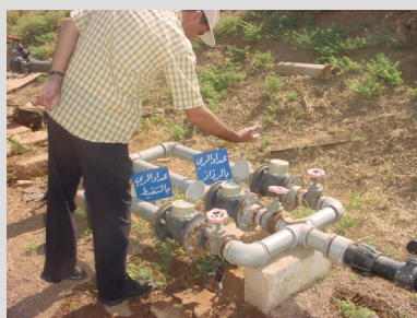
Flow meters equipped at the demonstration farm
